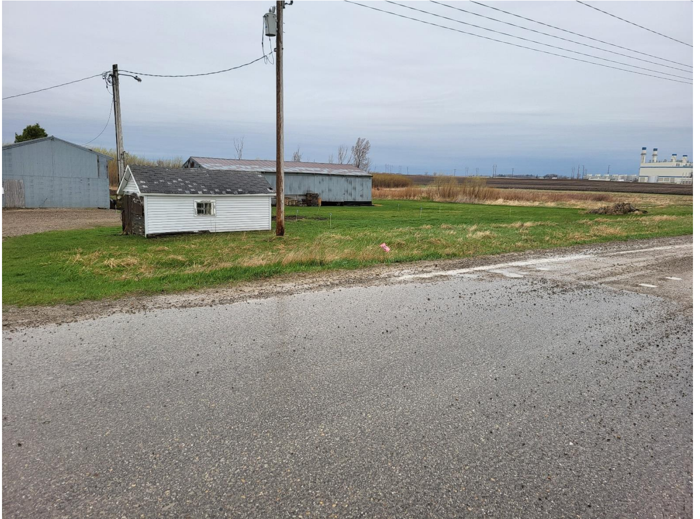
Figure 3 Looking southwesterly at building footprint from 230 th St
