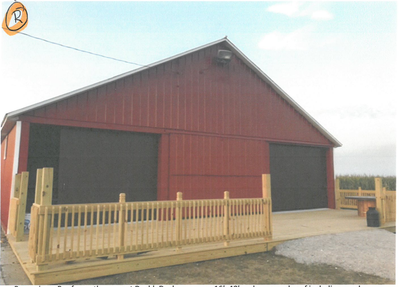
Proposing a Roof over the current Deck! Deck measures 16'x48' and proposed roof including overhang to be 18' x 50'! We want to do this to add shade!
