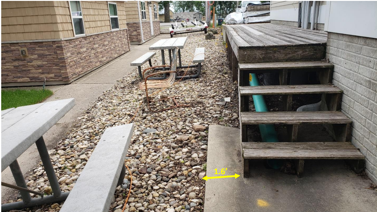
Figure 6 Looking southerly along the east side lot line
