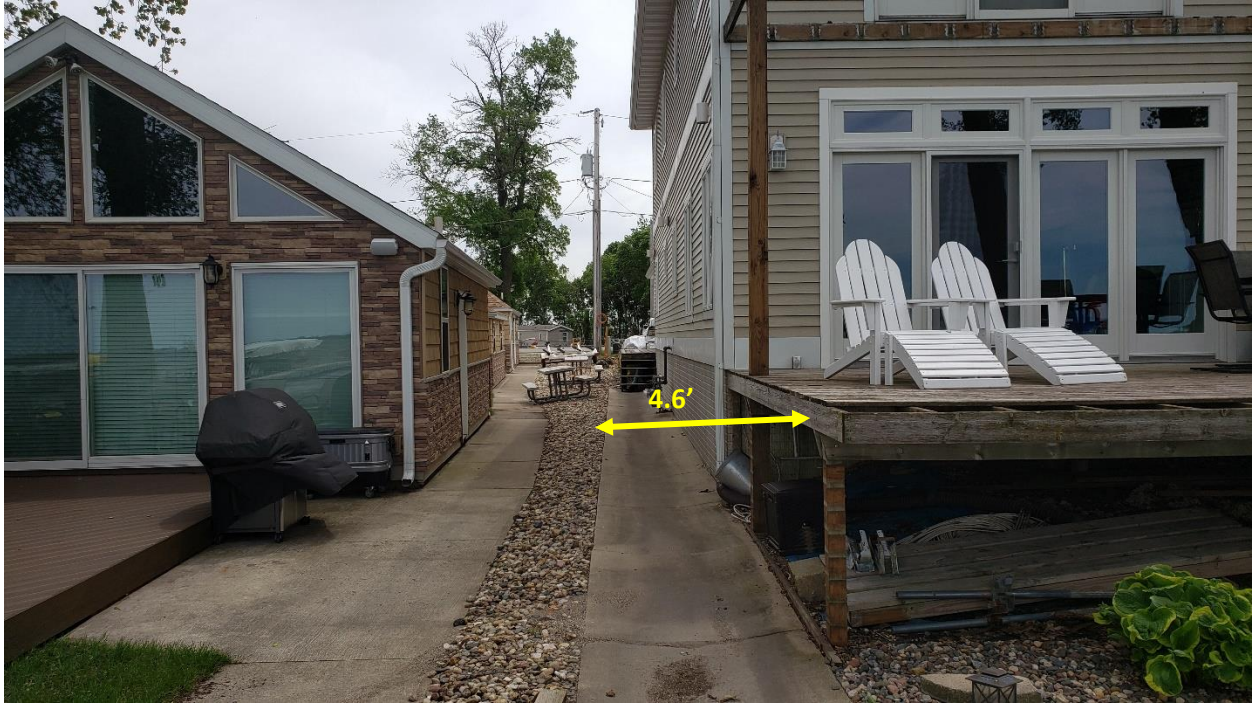
Figure 5 Looking southerly along the east side lot line
