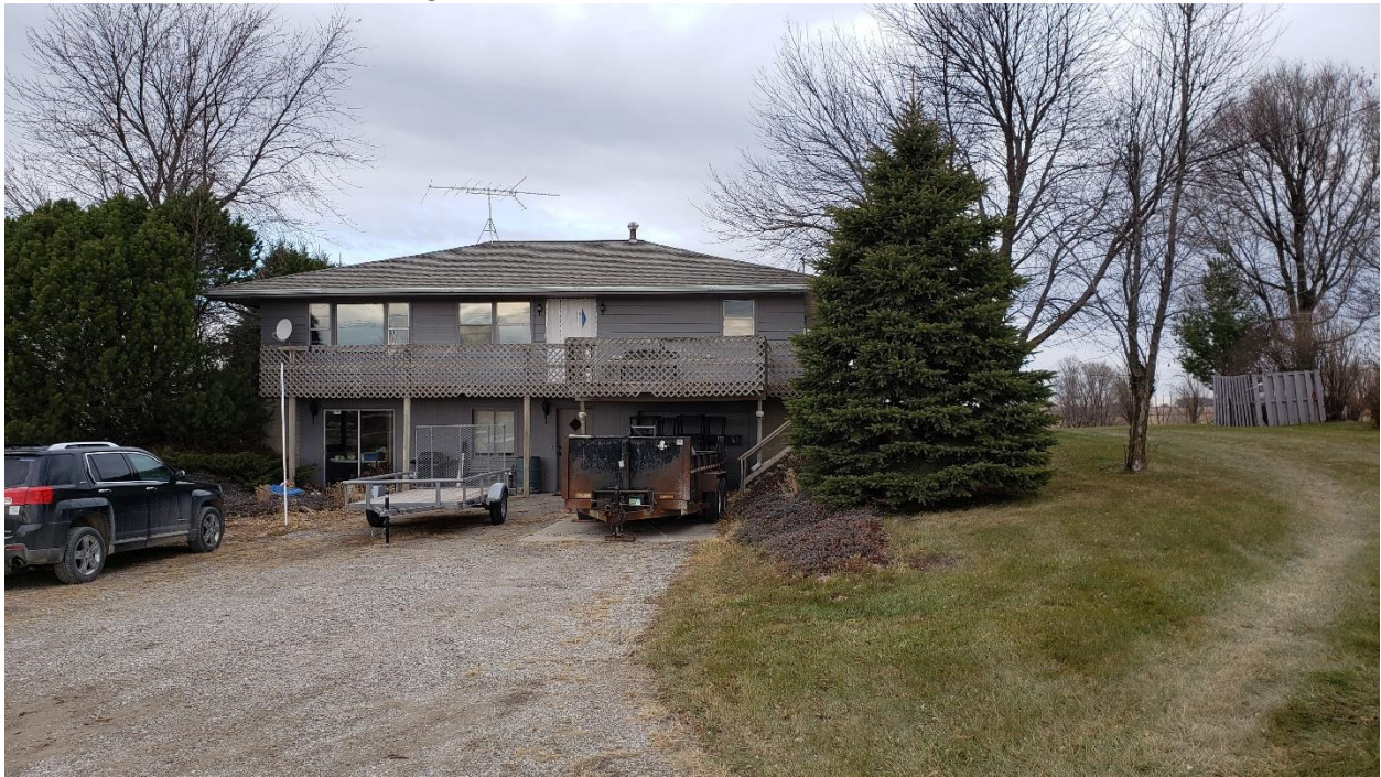
Figure 4 Looking at the Neve residence at 19288-A 290 th Street
