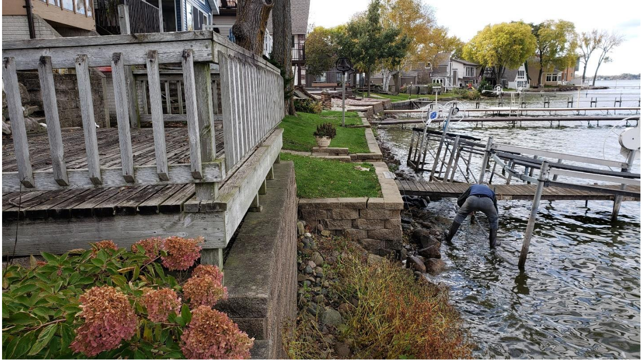
Figure 5 Looking west along the rear lot line
