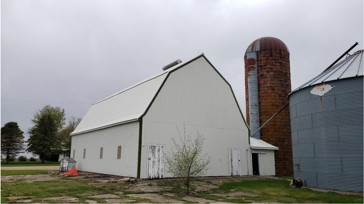
Figure 3 Looking at the easterly barn and silo
