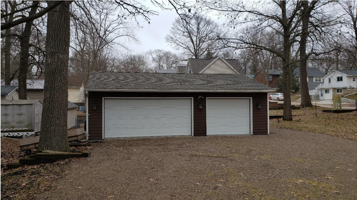
Figure 1 Looking at the existing garage
