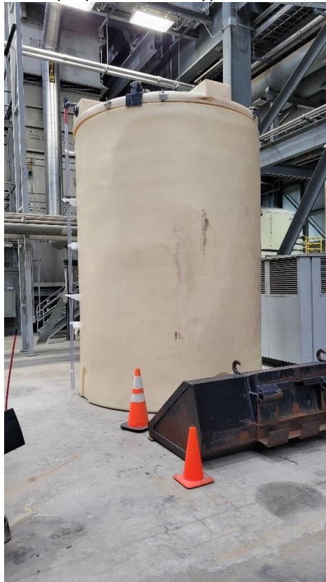
Figure 2 Looking at the proposed 6,550 hypochlorite storage tank
