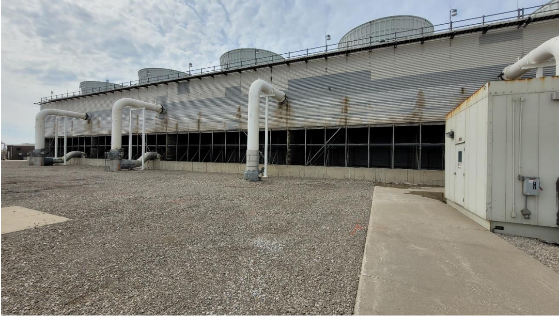
Figure 1 Looking at the proposed location for the new storage tank building
