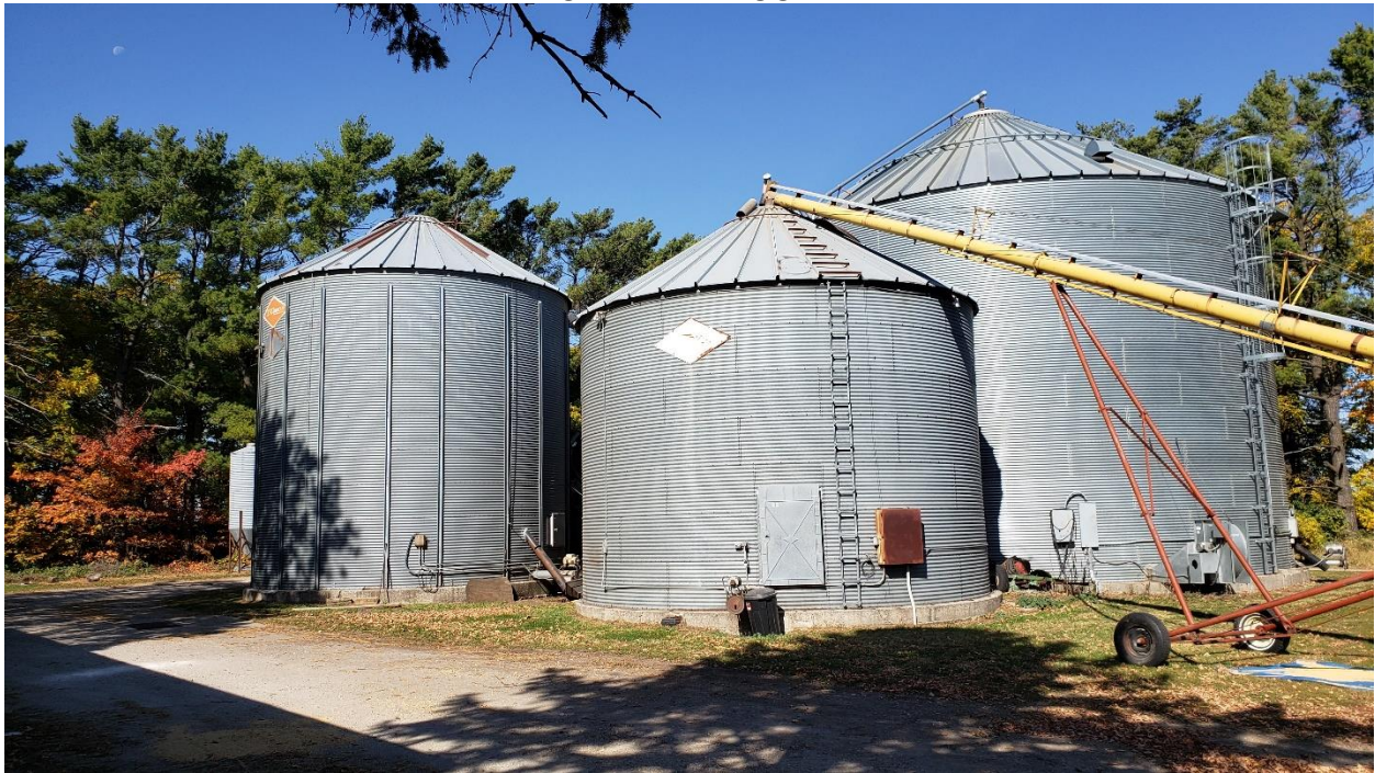
Figure 4 Looking at the existing grain bins
