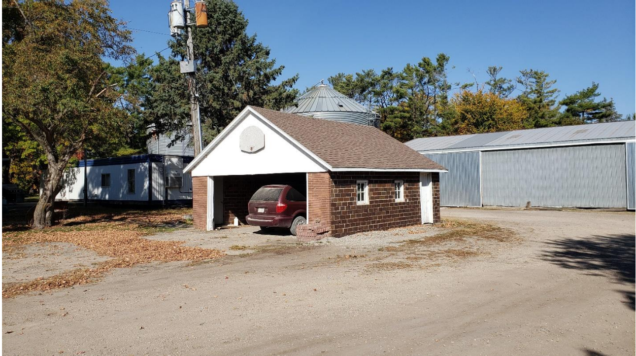
Figure 3 Looking at the existing detached garage
