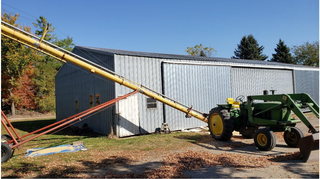
Figure 5 Looking at the existing machine shed
