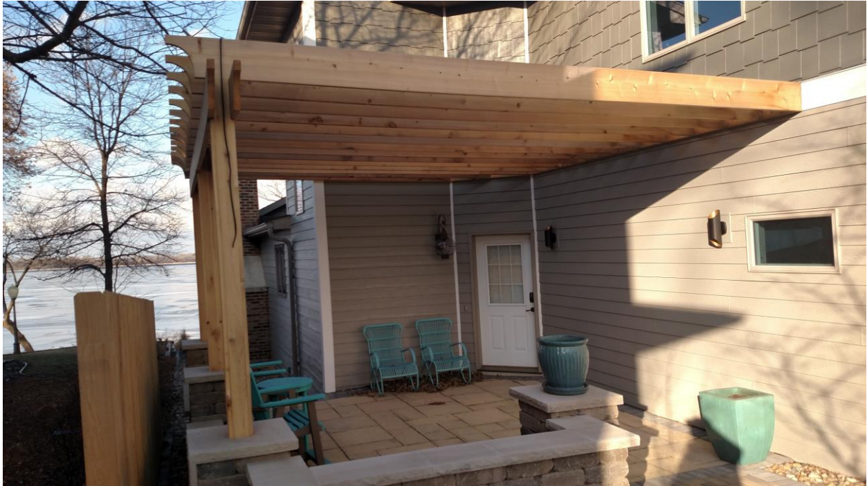
Figure 1 Looking at the pergola
