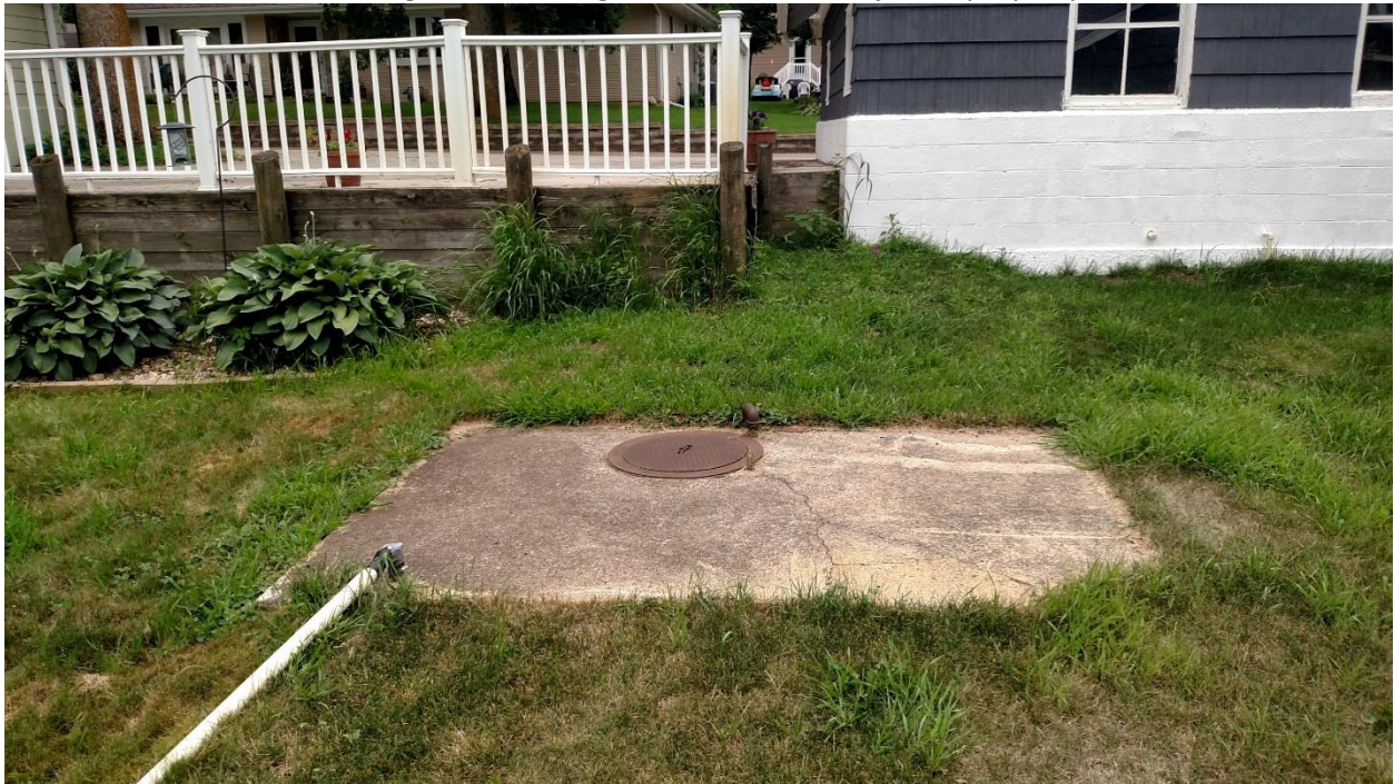
Figure 6 Looking at the drainage facilities on the adjacent property
